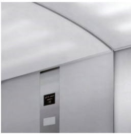
Ceiling: curved plexiglass and Neon lighting
